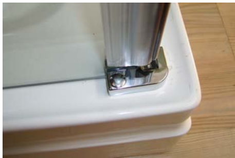
Zakrýt záslepkou cover with blind flange
