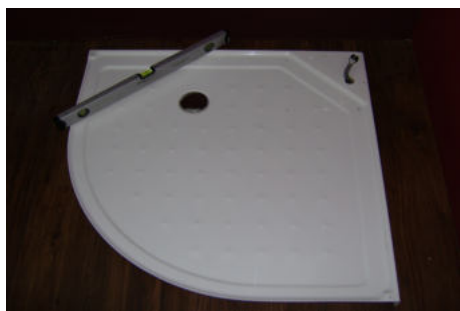
Vaničku ustavit do vodorovné polohy set the shower tray in horizontal position
